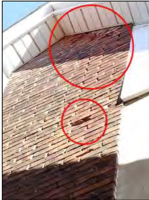
5. Masonry deterioration
