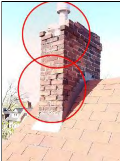
12. Loose, missing or deteriorated mortar
