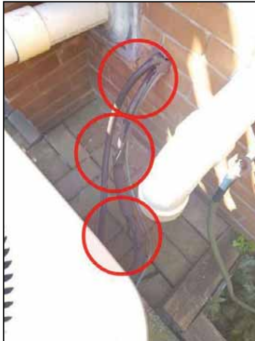
15. Insulation - missing
