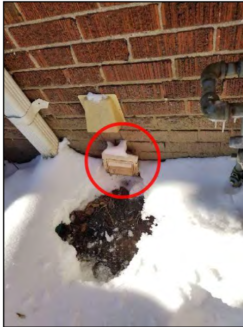
2. Cover damaged
