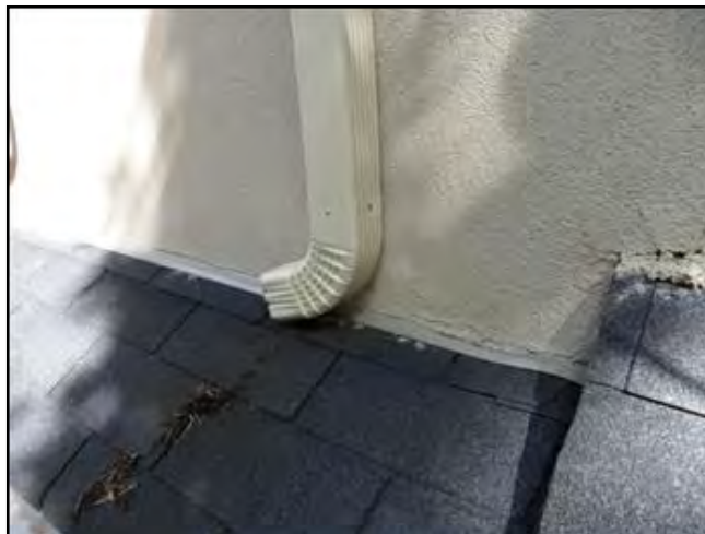
Discharge onto roof - extend to lower...
