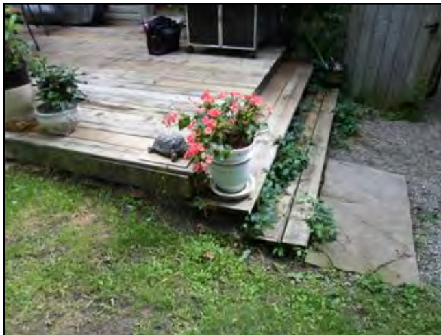
Ex : Wood-soil contact
