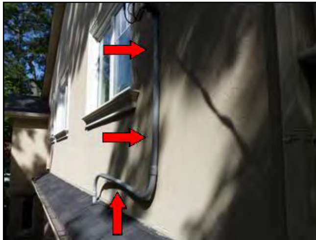
Mast clamps - missing/damaged/loose
