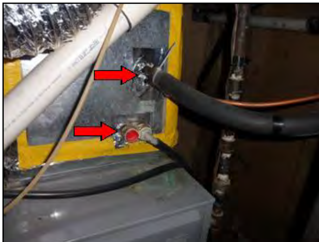
Unsealed gap at plenum
