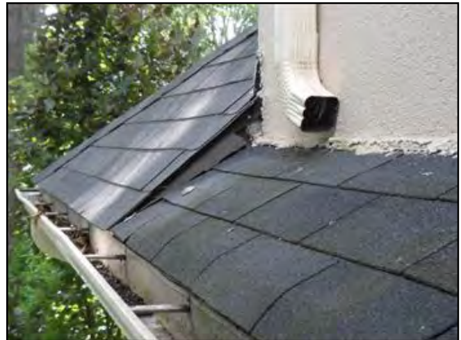
Counter flashing - missing or ineffective
