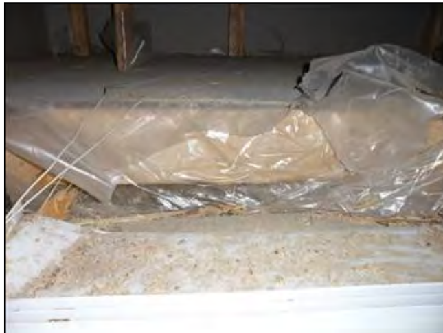
Concrete Formwork - not removed
