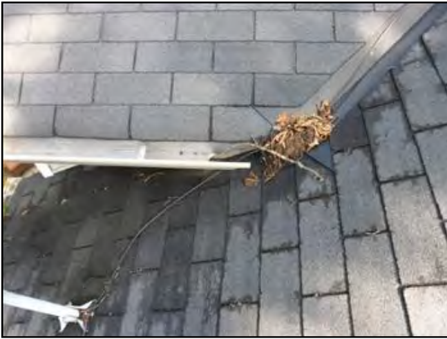
Discharge onto lower roof - causes...
