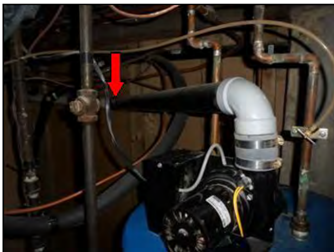
Exhaust Piping - slope suspect
