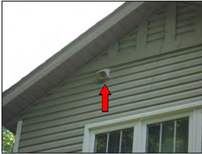
Vent Cap - suspect, loose
