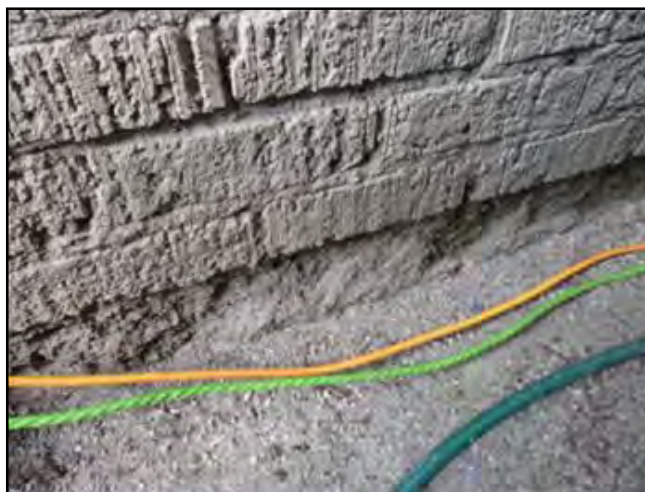
Ex: Freeze / thaw damage (spalling)
