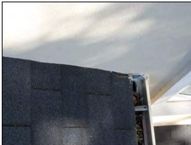
Kick-out flashing missing or ineffective
