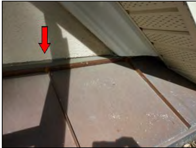
Caulking deteriorated/missing
