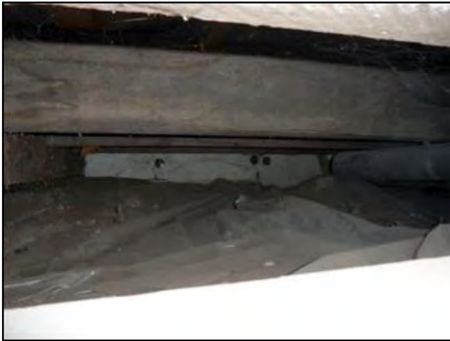
Restricted access (inadequate clearance)
