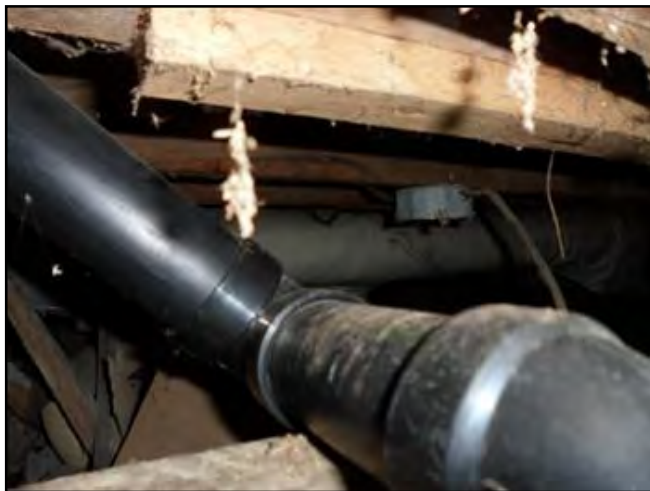
Restricted access (inadequate clearance)
