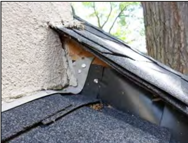
Counter flashing - missing or ineffective
