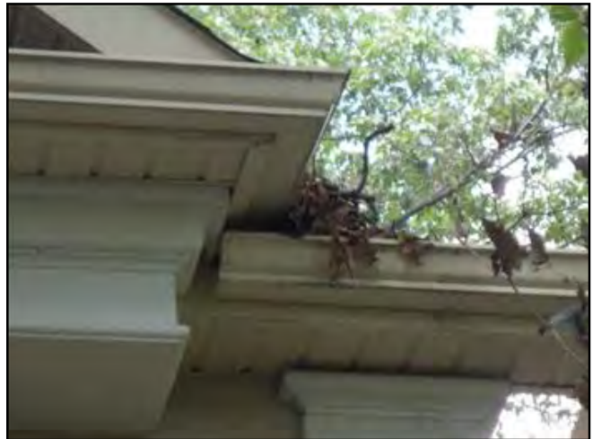
Discharge onto lower roof - causes...
