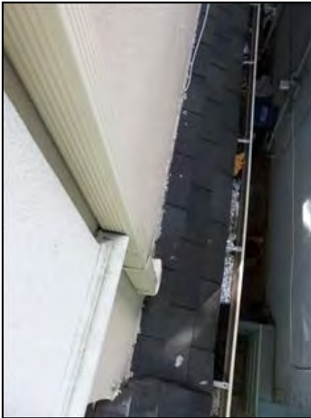
Discharge onto roof - extend to lower...
