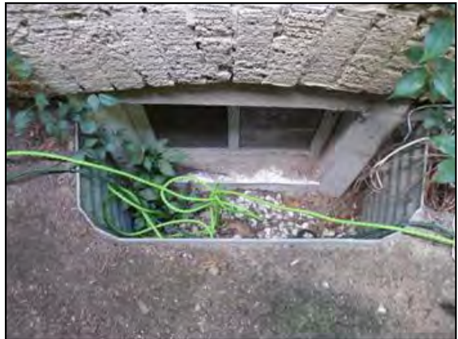
Window well - missing 6 to 8 inches...
