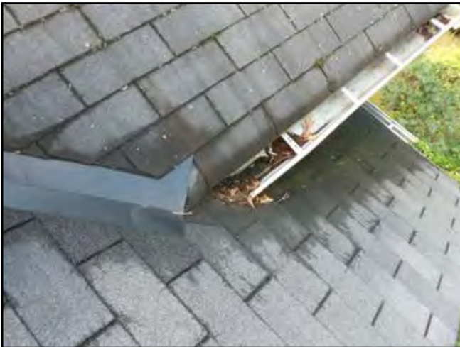
Discharge onto lower roof - causes...
