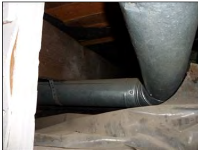
Restricted access (inadequate clearance)
