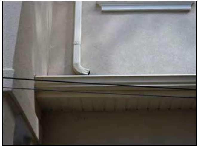
Discharge onto roof - extend to lower...
