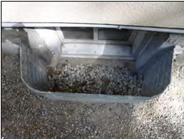
Window well - missing 6 to 8 inches...
