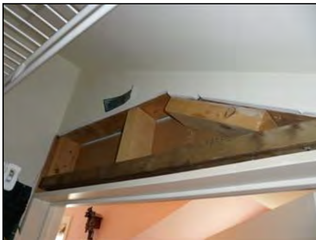
Drywall - installation incomplete
